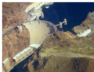
2 GIGAWATTS = 2,000,000,000 WATTS Peak output of the Hoover Dam
